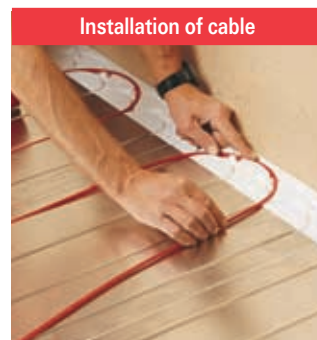
The T2Red heating cable is placed into the grooves. The desired heat output is determined by how closely you lay out the loops of the cable.
