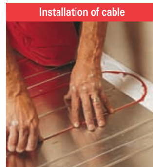
The T2Red heating cable is placed in the already prepared grooves of the plate. The desired heat output is determined by how closely you lay out the loops of the cable.
