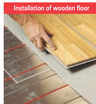
Place grey rag cardboard or foam on top of the Reflecta sheets and then lay the new wooden or laminated floor according to the instructions of the manufacturer.
