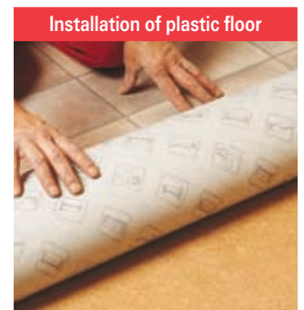
If the new overfloor is a plastic floor covering, first lay a 6 mm masonite or particle board floor on top of the grey rag cardboard or the foam, and then lay out the plastic carpet according to the manufacturers instructions.
