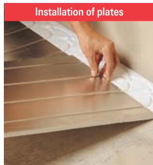
The Reflecta sheets may be glued to the underlying floor...
